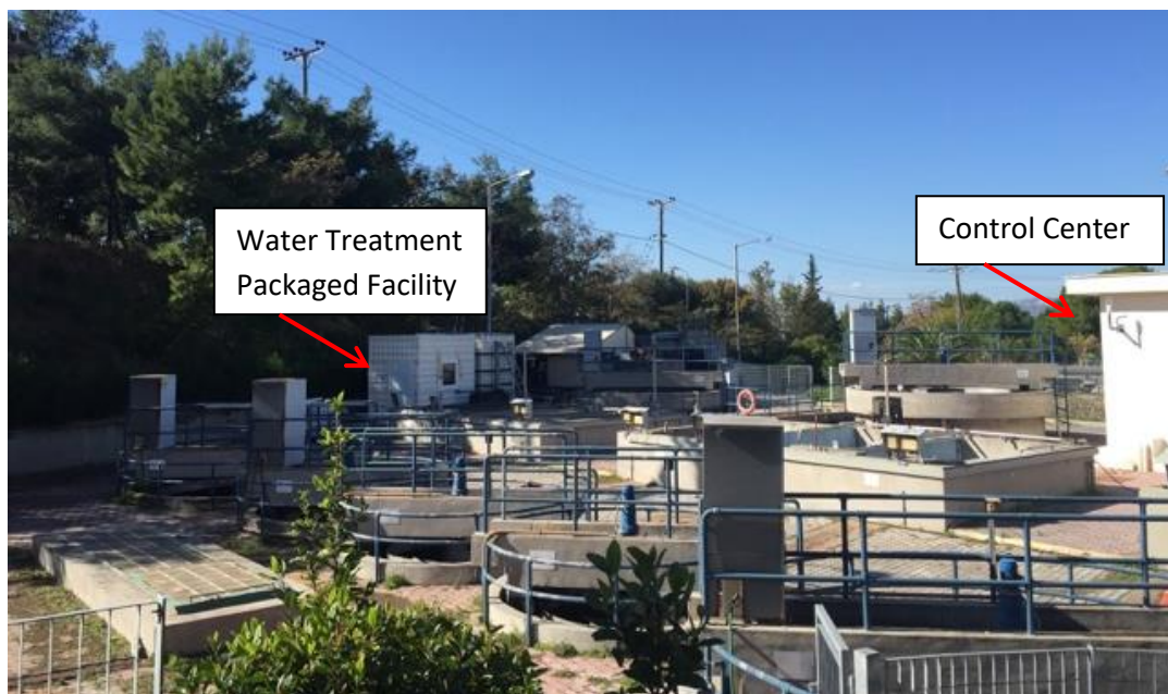
Figure 10: Athens KEREFYT Pilot Site – 2 (Overview)
